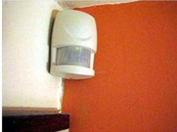
**The passive infrared (PIR) motion detector is one of the most common sensors found in household and small business environments.** It offers affordable and reliable functionality. **Passive refers to the fact that the detector does not generate or radiate its own energy** - it works entirely by detecting the heat energy given off by other objects.
